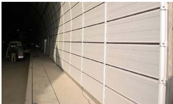
Modular Noise Barriers for High Speed Railways. Product installed and FEA Model of system components.
