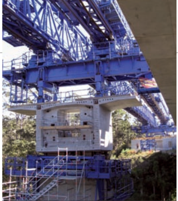
Above: Segments being lifted on the F11 Hunter Expressway project in Australia Below: Screenshot of the Geocon module
